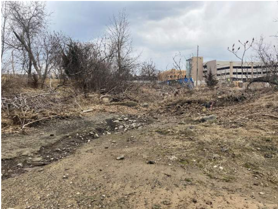
Photo 14 – Eroded channel in mitigation area at outlet of drainage swale (to be eliminated), looking south at approximate low tide. Taken 3/20/24
