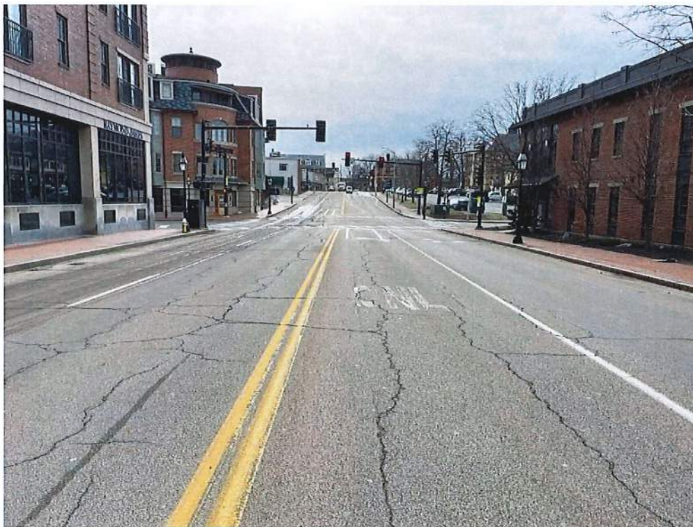
Photo 16 – Maplewood Ave between Hanover Street and Deer Street looking southeast. Taken 1/19/23
