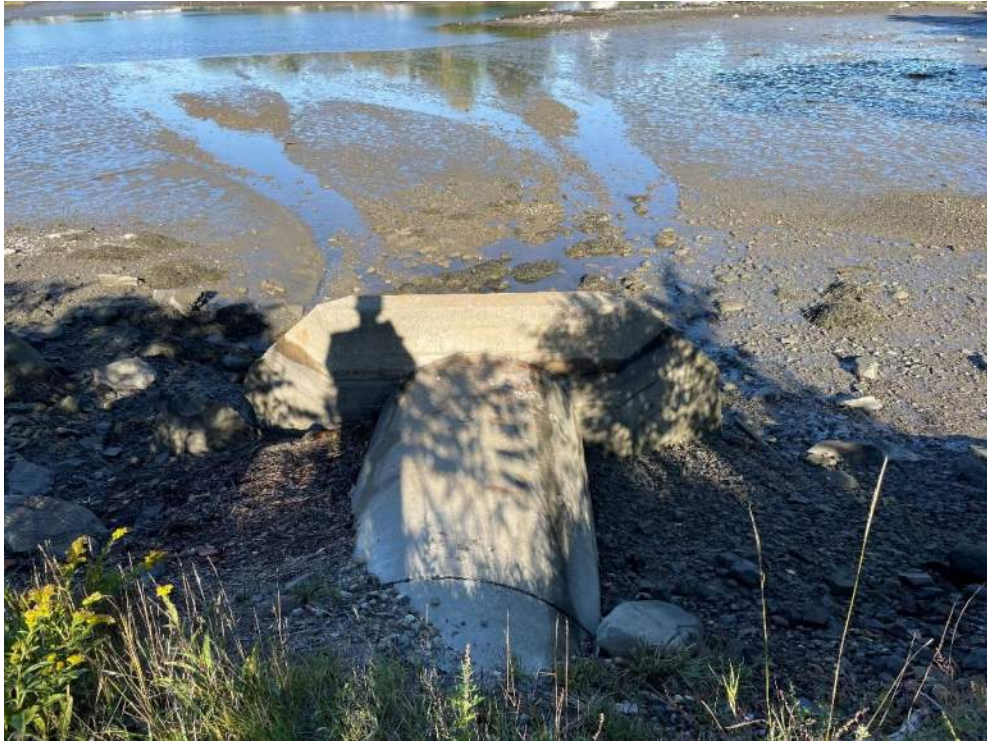
Photo 5 – Existing outfall headwall and exposed 48” RCP pipe looking northwest at approximate low tide. Taken 9/29/22
